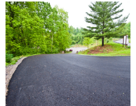
New entrance paving
