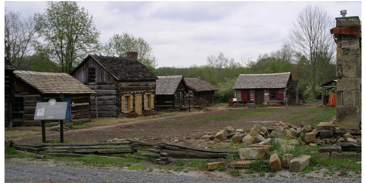
The commons as seen following the drainage installation.
