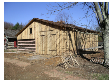
Side view of new Blacksmith Shop
